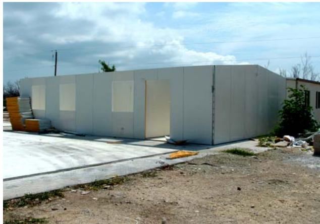
Picture of Unit with no roof, doors or windows
