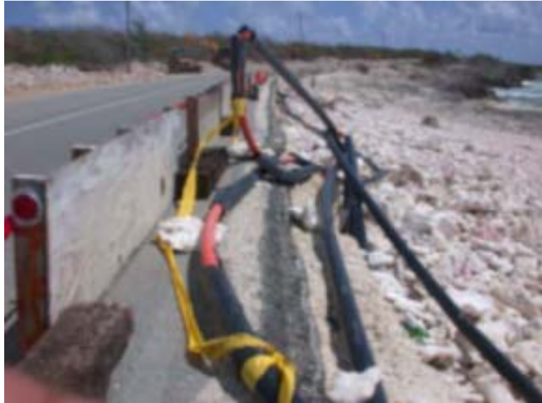
Figure 3.8 Fibre-optic cables exposed by erosion of the south coast road.
