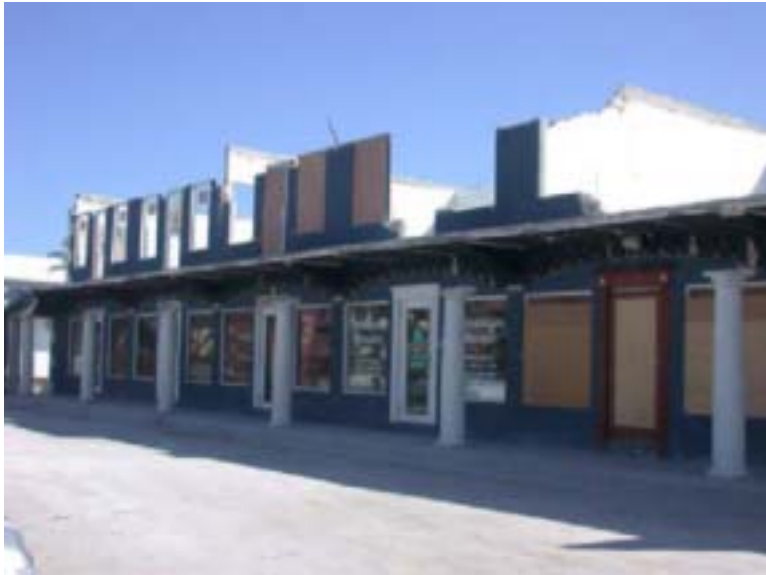
Figure 3.3 Severe damage to the upper level of a pre-code un-reinforced masonry building by wind during Ivan.
