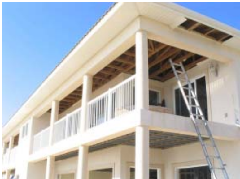
Figure 3.4 Boxed-eave coverings suffered extensive damage and allowed major water ingress to many residential and hotel properties.
