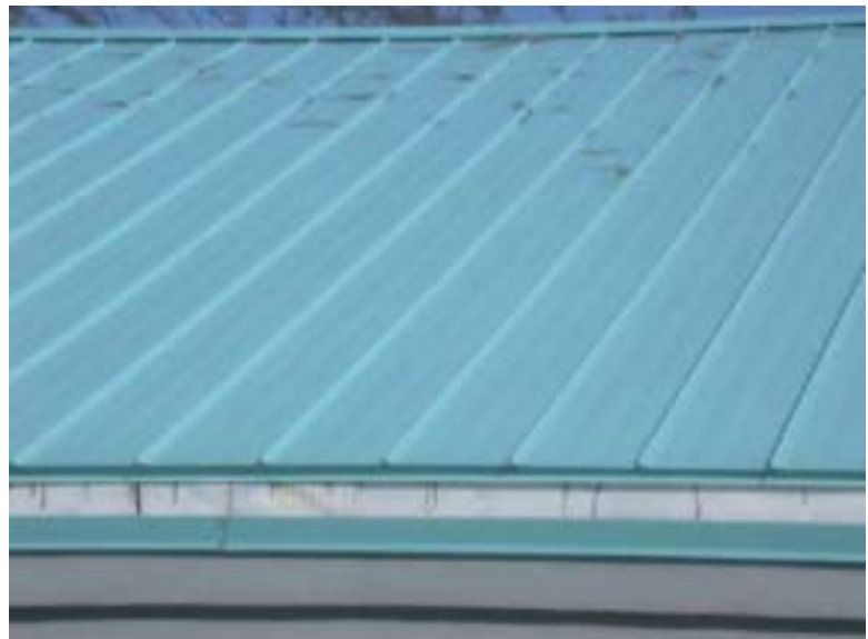
Figure 3.23 Standing seam roofing did very well in Ivan.
