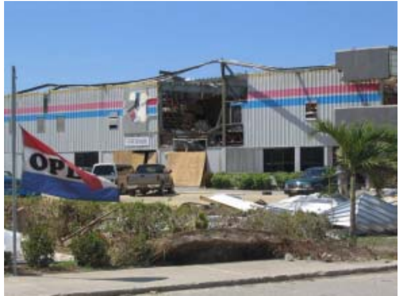
Figure 3.30 Long-span galvanised siding blown out and subsequent loss of a large part of the building.
