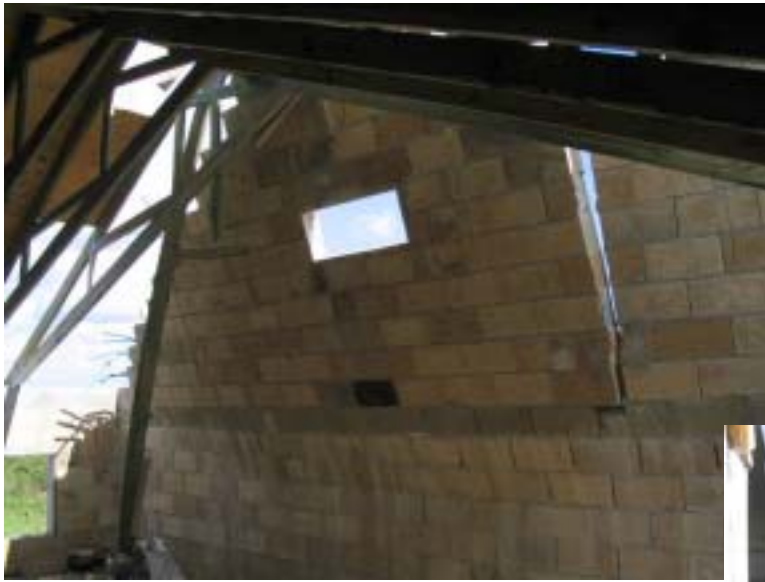
Figure 3.24 Compromised gable end in a house under construction.
