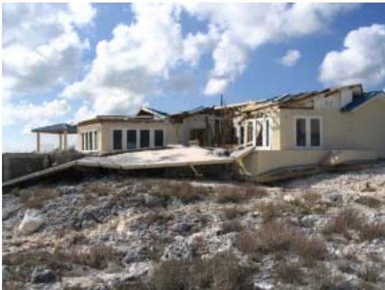
Figure 3.26 Extreme wave damage at High Rock; this property is about 25 ft above sea level and several hundred feet from the shoreline.
