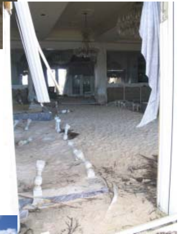
Figure 3.25 Ingress of sand and flood water was very severe in many areas along the south coast beaches. This property is in Bodden Town.
