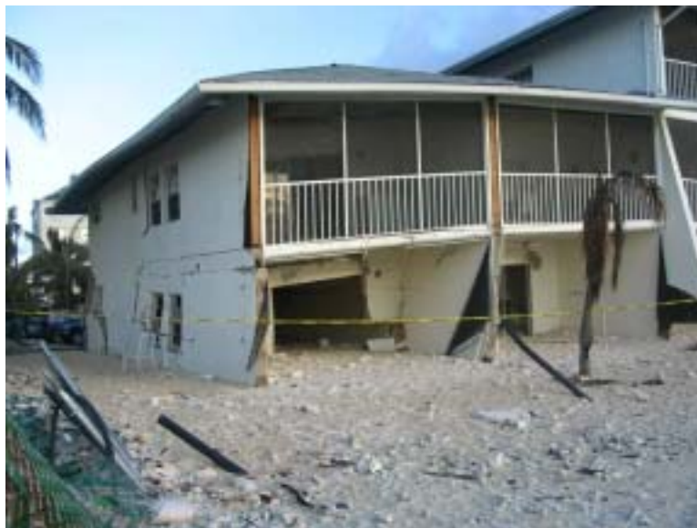
Figure 2.11 Damage at this location on Seven Mile Beach was due to erosion by fast-moving storm surge flood water confined to a narrow passageway between buildings.
