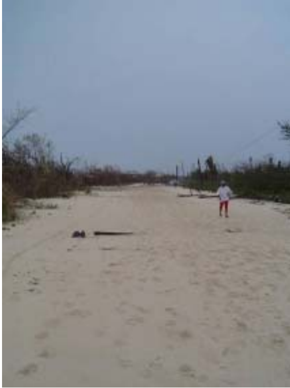
Figure 3.6 West Bay Road adjacent to Seven Mile Beach, where storm surge flooding carried and deposited sand across the roadway.
