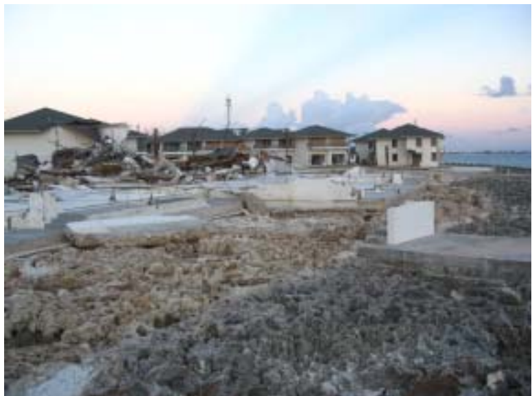
Figure 3.19 Dolphin Point, West Bay. Onshore winds late in the storm drove heavy waves into this and adjacent properties, causing massive damage, even to well-built reinforced masonry structures.
