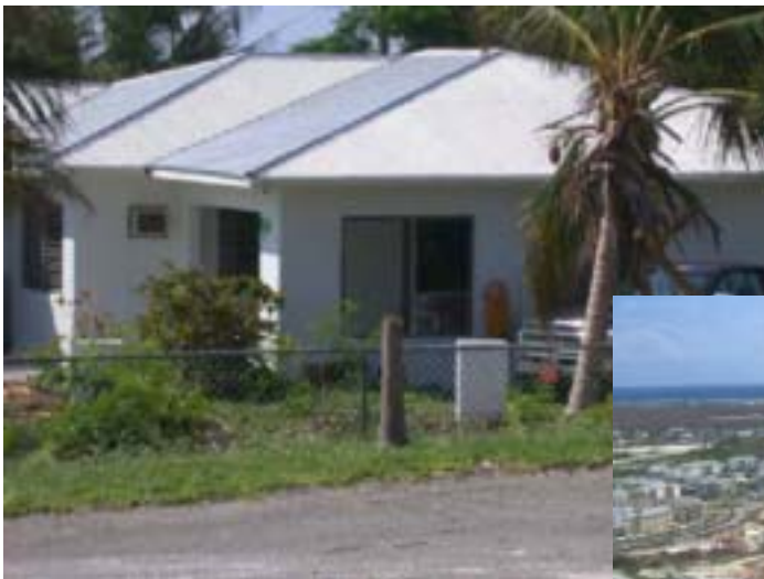
Figure 3.20 Traditional arc-tangent roofing fared well in Ivan, much well-installed roofing cover remaining fully intact.
