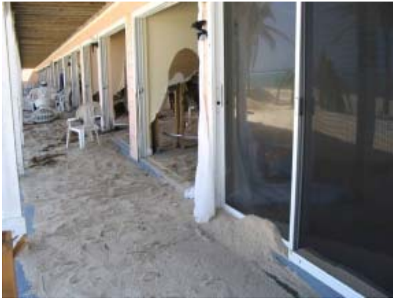
Figure 3.15 Storm surge flooding caused extensive damage to ground floor rooms in most beachside properties around Grand Cayman. This is the Morritt's Tortuga Club at the north end of the east coast.
