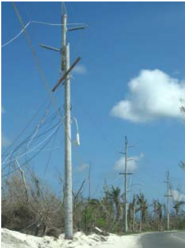
Figure 3.11 Failure of concrete pole at a bolting point. Along south coast road near Bodden Town.
