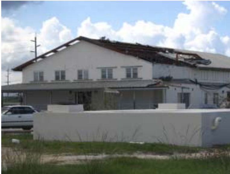
Figure 3.32 Extensive roof damage at Bodden Town Civic Centre, which at the time was being used as a shelter.
