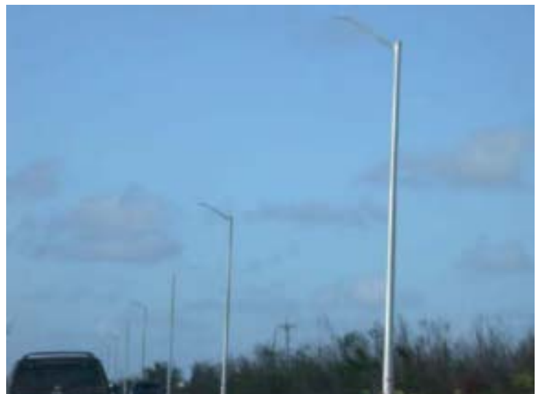
Figure 3.13 Street lights lost from stand-alone poles.
