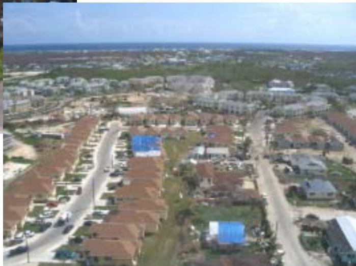
Figure 3.21 New housing in Windsor Park, George Town. Most of the asphalt shingles stayed on despite the strong winds.
