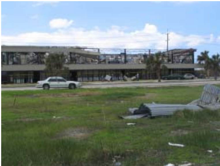
Figure 3.29 Loss of long-span galvanised roofing and subsequent destruction of the entire property was frequent around George Town.
