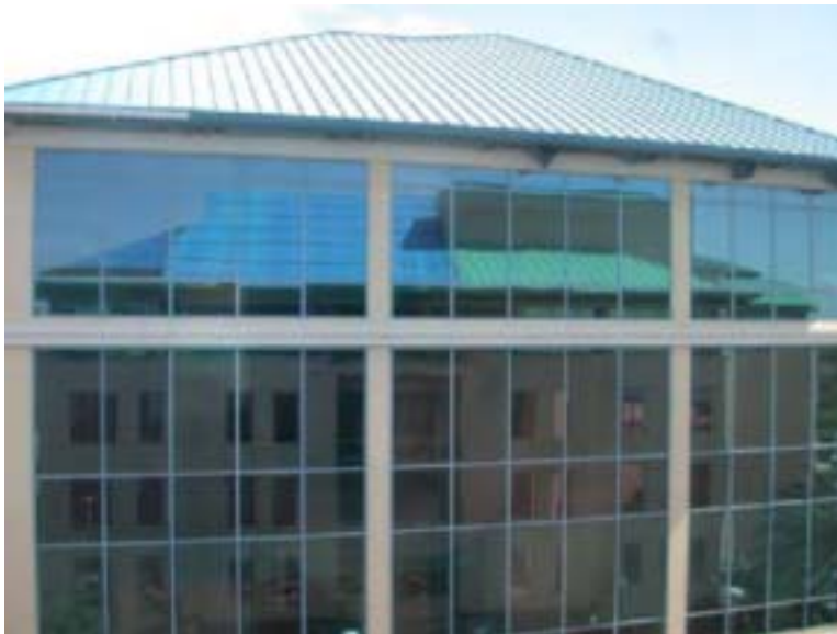
Figure 3.27 Laminated glass performed very well in office buildings throughout Grand Cayman.
