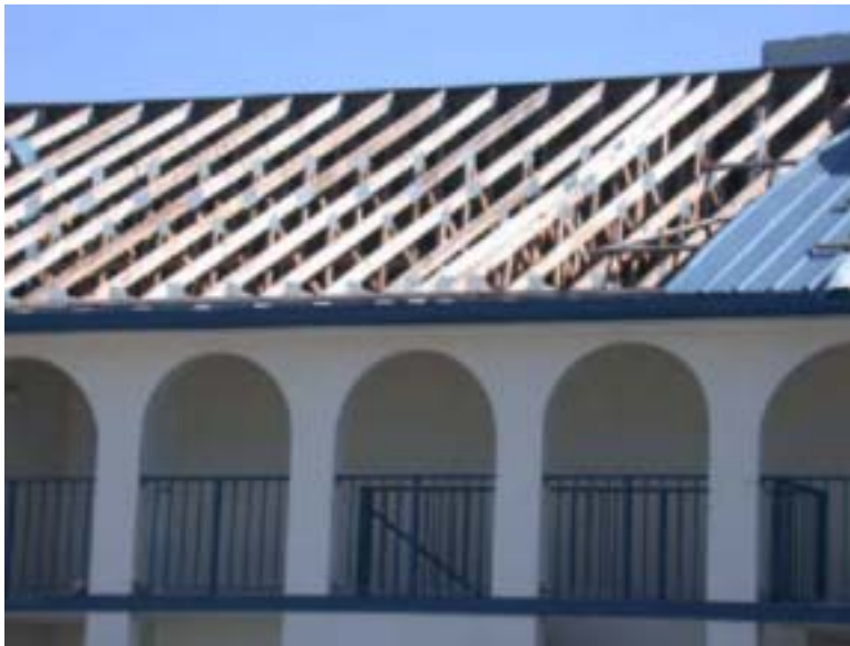
Figure 3.33 Galvanised connector plates on roof trusses kept the roof structure intact, although the roof covering was lost.
