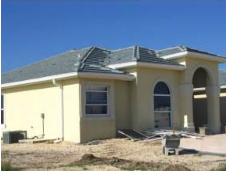
Figure 3.22 Clay tiles removed from the east-facing roof and from ridges on this house in Governor's Harbour.
