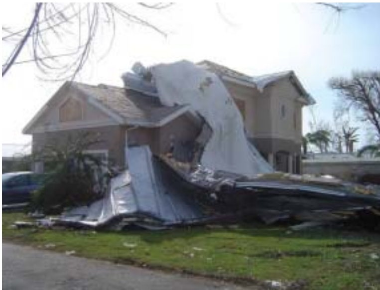
Figure 3.31 The roof from a neighbouring building caused significant damage to this otherwise well-protected residential home.
