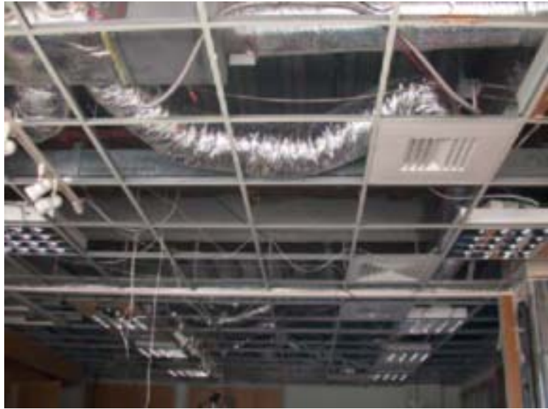
Figure 3.28 Significant internal damage was caused by rain ingress through minor breaches in the building envelope.
