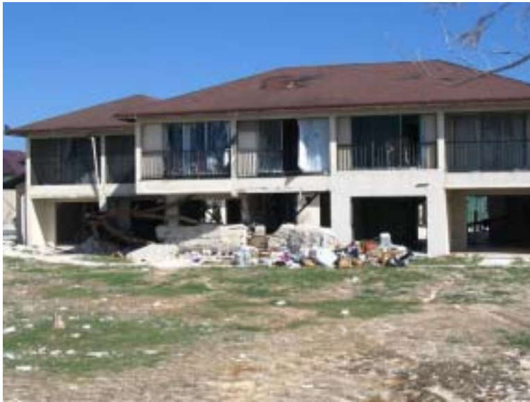
Figure 3.18 Ocean Club along South Sound; next door, the wooden structures of Mariner's Cove were completely destroyed. Note parts of the sea wall used as a battering ram causing severe structural damage.
