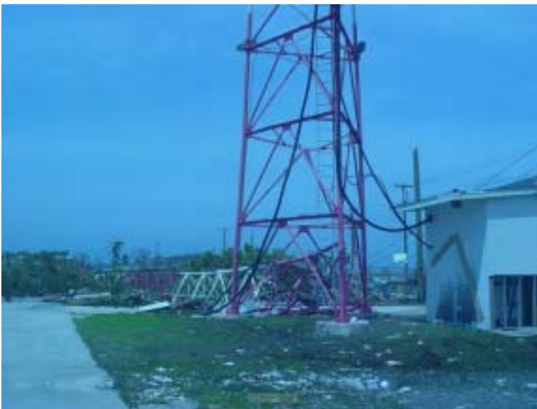
Figure 3.7 Upper segments of tall communications tower blown off by Ivan
