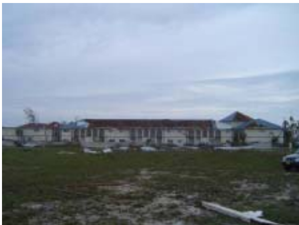
Figure 3.17 (below) Major roof covering damage to Indies Suites on West Bay Road (left) and minor damage to the much newer Morritt's Tortuga Club (right).
