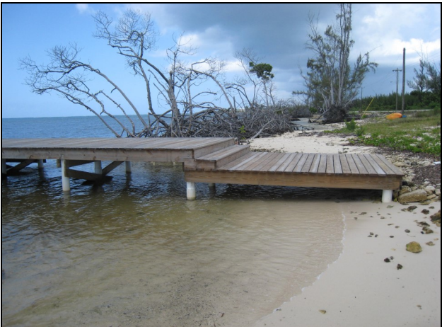
Photo 1: Good example of a dock design which does not block pedestrian access between the low and high water marks.
