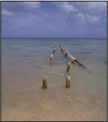
Photo 4: Removal may be necessary if a damaged dock is creating a navigational hazard. The Port Authority can advise on this. A Coastal Works Permit is required for works on the seabed.
