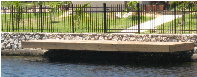
Photo 2: The above dock is cantilevered from the canal wall and therefore does not require pilings. A similar technique should be used for swim and fish cleaning platforms on ocean front docks.
